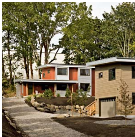
FAR LEFT Charlie Weiss and Katharine Lawrence’s green home has an impressive plumbing network (affectionately called “the wall of wonder”) that not only filters rainwater, but also heats it geothermally and distributes it throughout the house.
