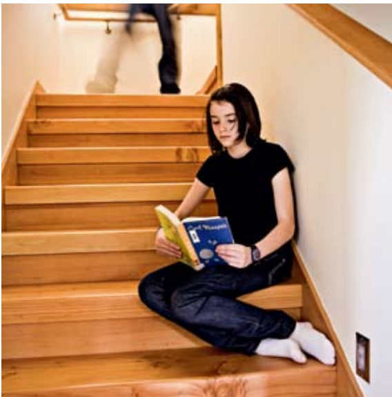
LEFT Leapfrog's interiors showcase sustainably harvested and reclaimed wood products, including trim milled from old high school bleachers (above) and elegant stairs cut from a fir tree felled on site (below).
